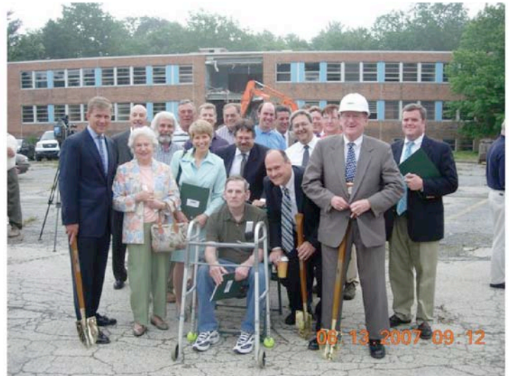
June 13, 2007 Ground Breaking and beginning of demolition: Front row left: Commissioner Andy Lewis, Lucetta Alderfer, Grant project volunteer; Jan Marie Rushforth; Chair Ad Hoc HSH Board; Wilbur Clevens, Park & Rec Board; (behind wheelchair) Commissioner Tom Broido, (kneeling) Commissioner President Steve D'Emilio, Commissioner Jim McGarrity, Row behind: Bob Freedman, Goldenberg Group; Todd Pohlig, Pohlig Builders; George Rementer, Finance Director Haverford Twp; Brian Barrett, Park & Rec Program Director and Ad Hoc HSH member; Dr Joe Martin, Grant project and School Board Director; Tim Denny, Assistant Township Manager and Park & Rec Director; Commissioner Mario Oliva; Rich Caroto, Chair Park & Rec Board; David Brooman, Township Attorney on HSH; Peter Hickman, Grant project and Ad Hoc HSH Board, and Commissioner Larry Holmes. Photo taken by Jean Marie Lorello.
