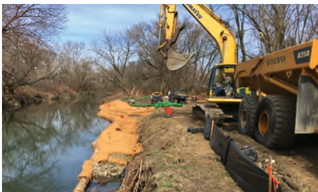
Figure 1-2. US EPA provided photo of Mudsill during its construction along Darby Creek. Figure 3. US EPA provided photo of Mudsill after restoration planting has had time to grow.
