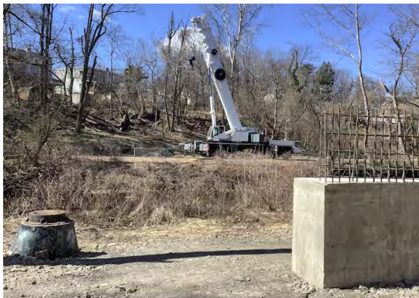
Crane to hoist bridge into place
