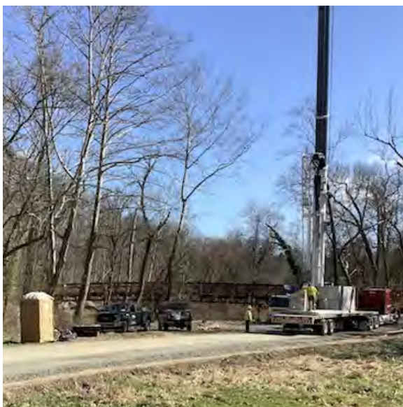
Bridge in place
