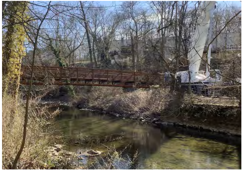
Bridge view from Swedish Cabin
