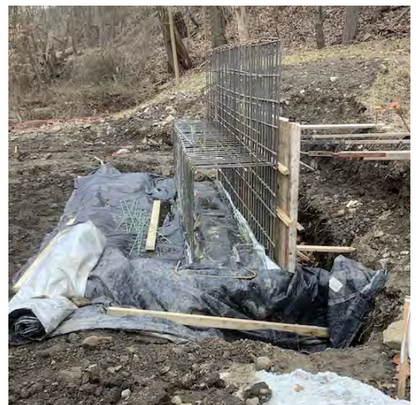
Rebar for abutment
