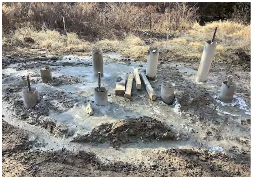
Micro piles to anchor the concrete
