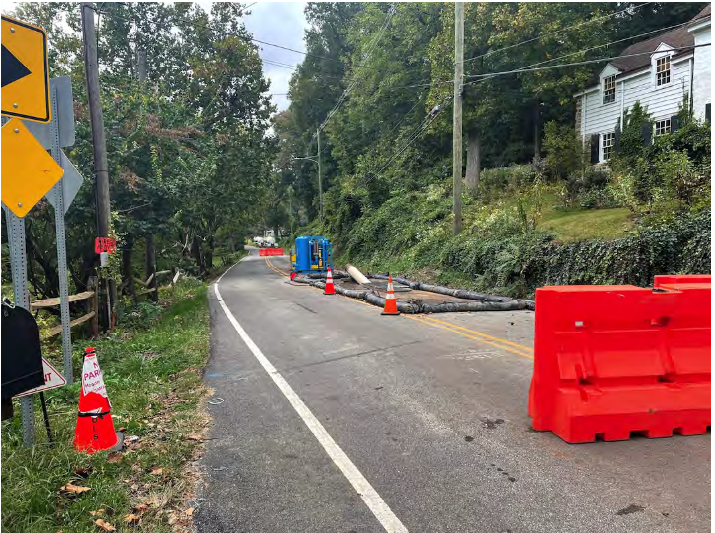
View from West (pipe emerging from pylons)
