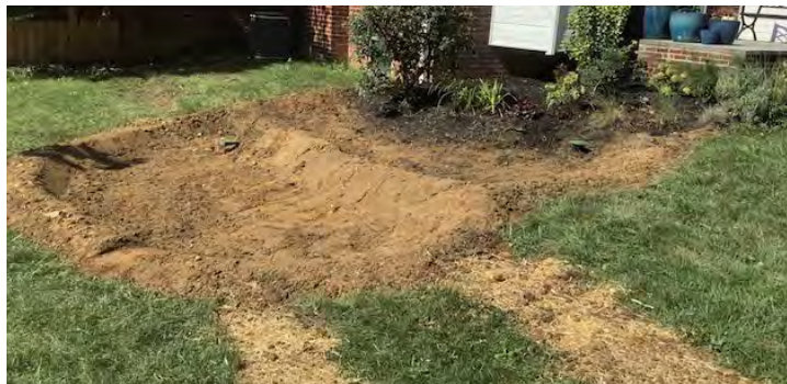
Excavation, berming and pop ups
